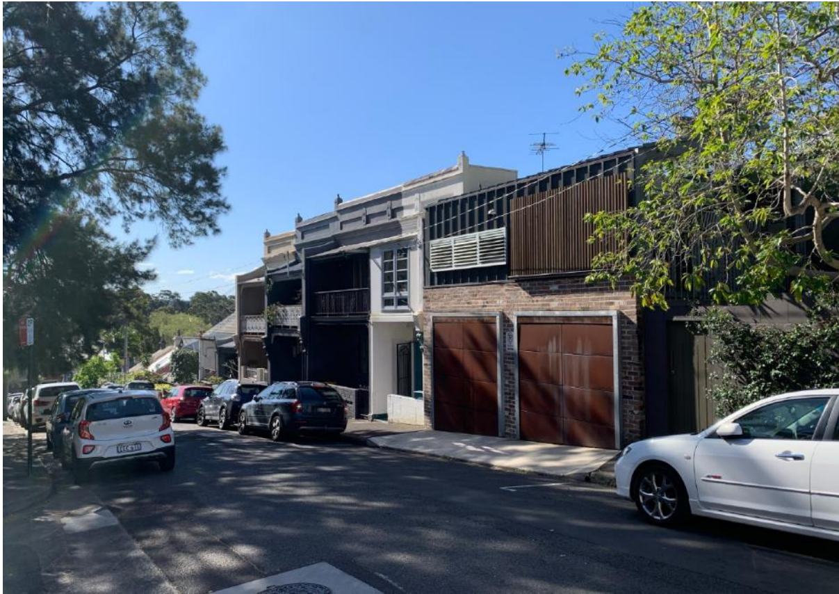
Figure 18: Avon Street terraces opposite the subject site
