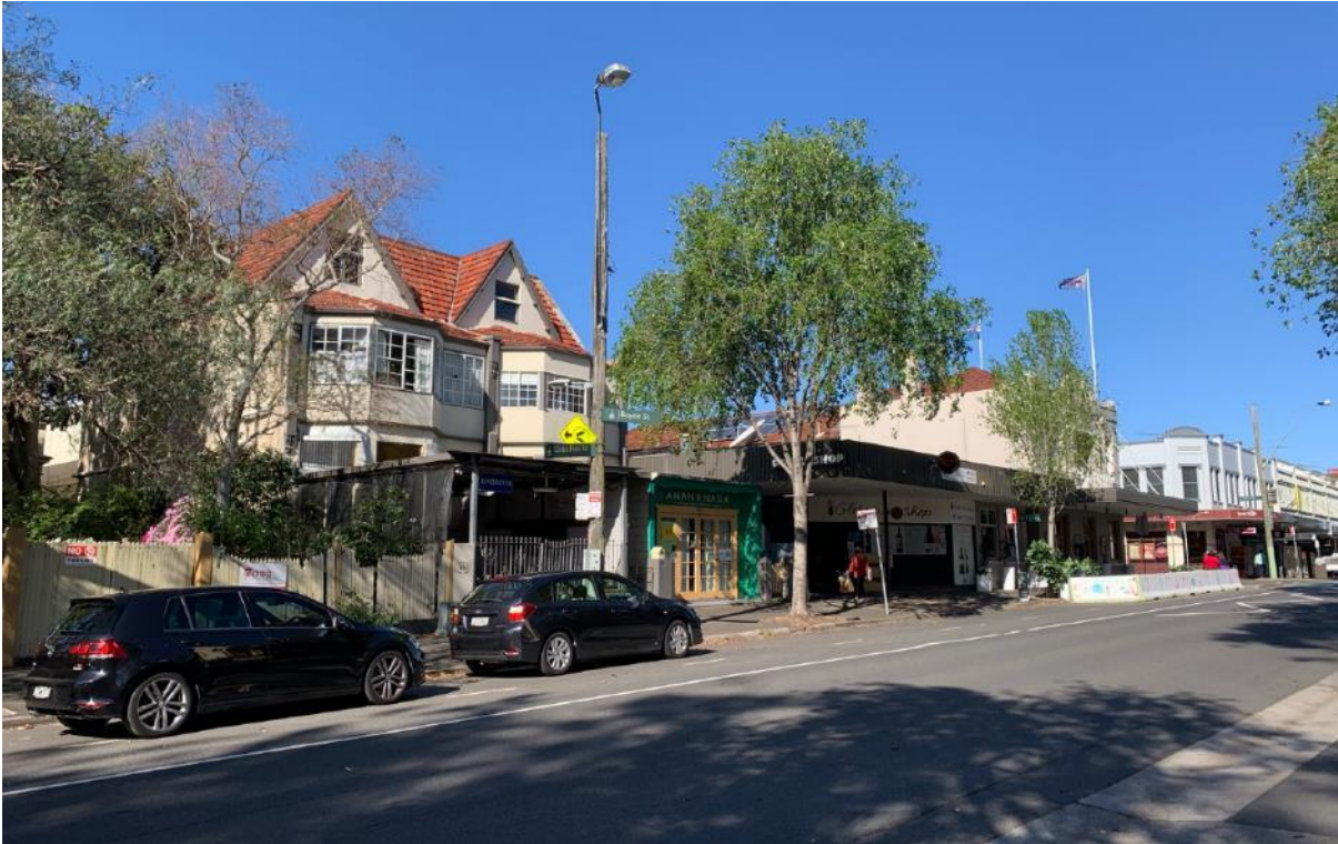
Figure 10: Adjoining commercial properties to the south on Glebe Point Road
