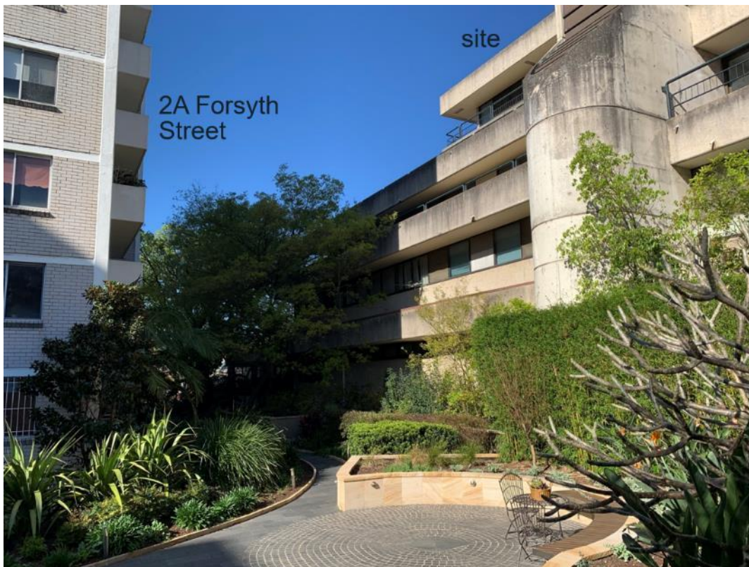
Figure 6: MRC building (north elevation) viewed from 2A Forsyth Street
