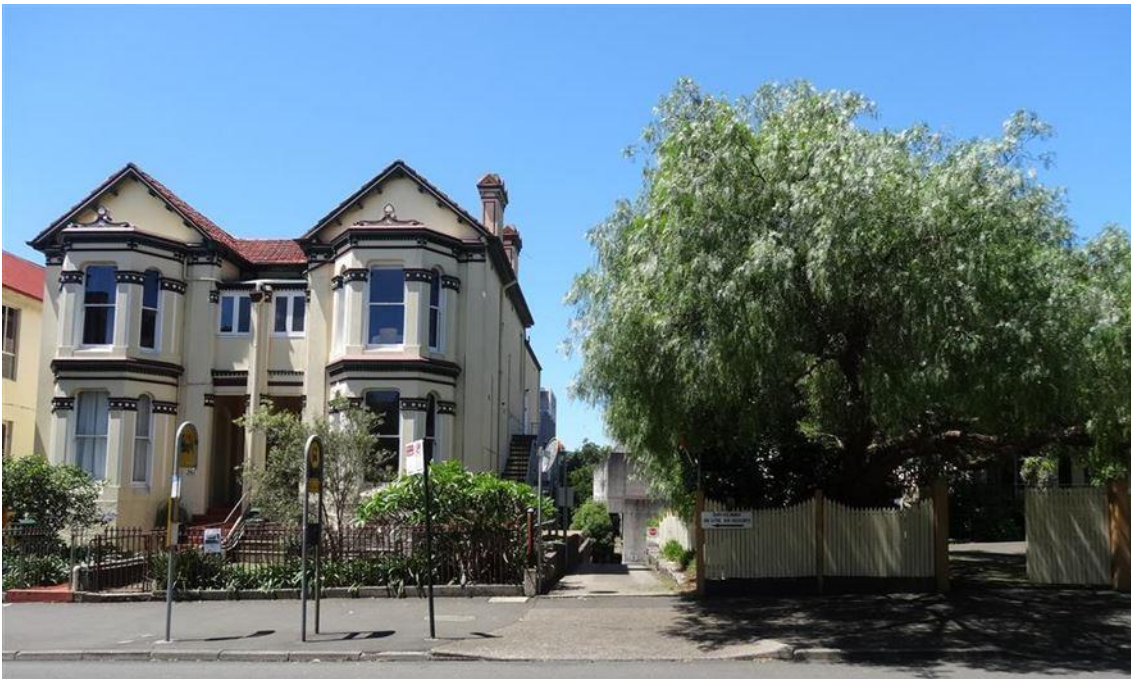
Figure 11: Adjoining two storey dwellings at 359-361 Glebe Point Road. Access to the basement of the MRC building from Glebe Point Road is at the centre of the image.
