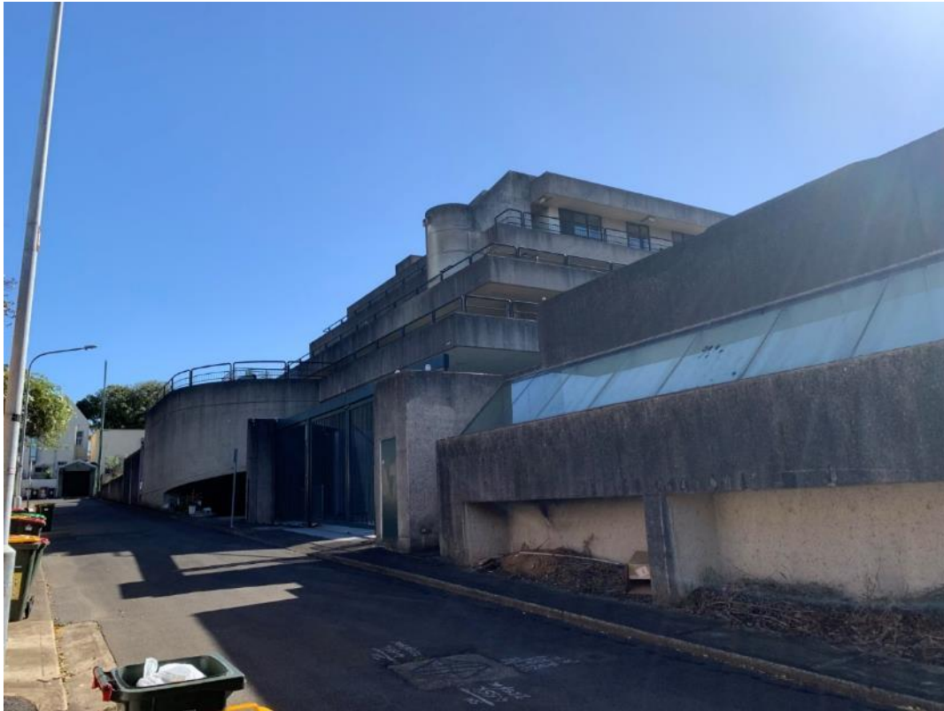
Figure 7: MRC building viewed from Ferry Lane (south elevation)
