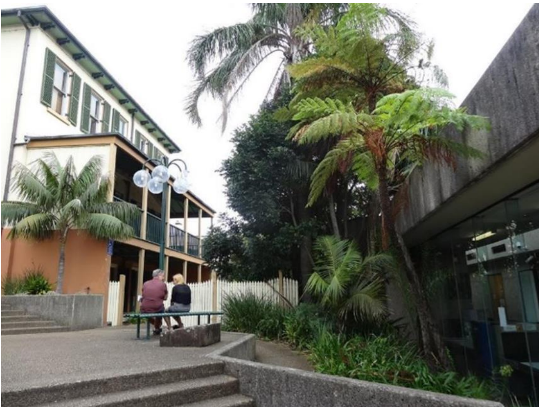
Figure 4: Rear of Bidura House (left) and existing relationship with the Metropolitan Remand Centre (MRC) (2017)
